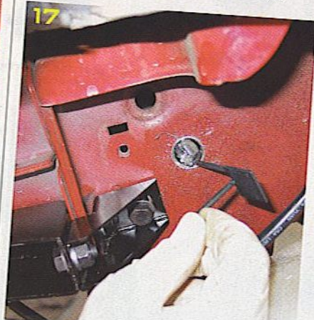
17. THE BRACKETS ARE THEN BOLTED BACK IN PLACE, BUT THE FASTENERS ARE ONLY MADE HAND TIGHT UNTIL THE REST OF THE MOUNTING HARDWARE CAN BE SECURED. THIS WOULD NORMALLY BE SOMETHING OF A CHALLENGE SINCE ONE OF THE MOUNTING POINTS IS ON THE FRAME RAIL AND THE OTHER IS ON THE BUMPER EXTENSION AND NEITHER SEEMS EASILY ACCESSIBLE FROM BEHIND. TO REMEDY THIS, KÖRBACH INCLUDES A COUPLE OF "STICK NUTS," NUTS ATTACHED TO SMALL METAL STICKS THAT ALLOW YOU TO FISH THE NUT BEHIND THE BOLT. FOR THE REAR BRACKET AN ANGLED STICK NUT PASSES THROUGH THE 5/8-INCH HOLE DRILLED EARLIER, WITH THE NUT LINED UP BEHIND THE MOUNTING BOLT AND THE BOLT TIGHTENED HAND TIGHT.
